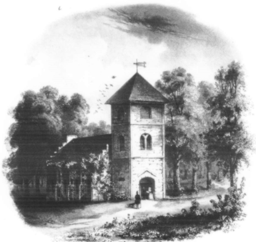
Defau's This Church near Smithfield, Isle of Wight Co. Va. built in the reign of Charles I st between the years 1620 & 1622.
